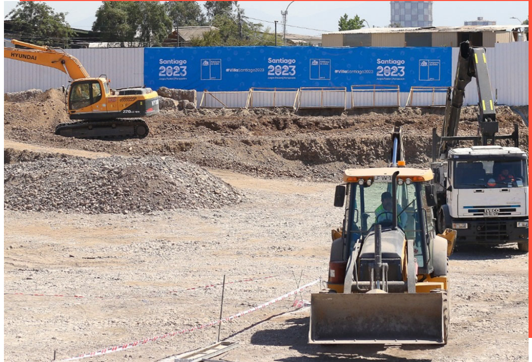
The construction works of the Pan American and Parapan American Village.
